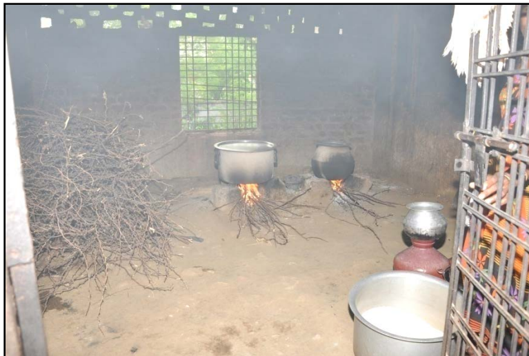
Kitchen Shed in the sample School
